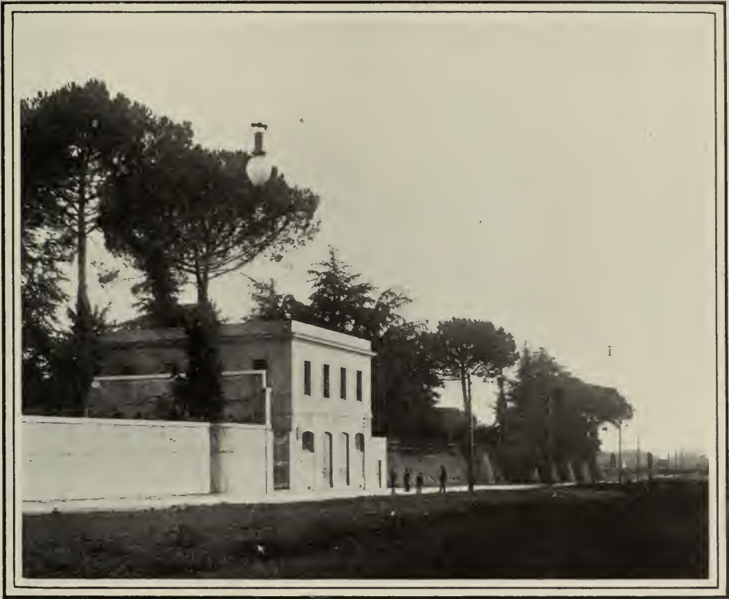
FIG. 7. THE PORTA PIA TRANSFORMER STATION.
